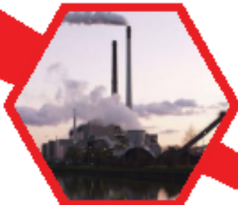
Coal Burning Utility
