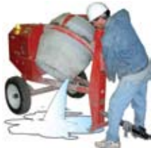
2 DO NOT drain into repair site!
