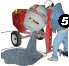
5 Mix for 6 additional minutes (7 minutes total) and place. Pour DOTline™ into repair site. Screed and finish DO NOT RE-TEMPER WITH WATER
